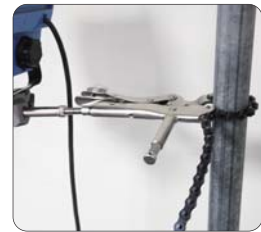
On the steel tube
